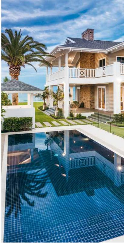
The property is located on a beachside block where units were originally situated, so the unit block had to be demolished and removed prior to the new construction. Due to the void that was created after demolition, the pool was fully-formed above ground, and a freestanding concrete structure was required. JB Pool Construction installed 20 steel screw piers to anchor the pool, as well as additional footings to suit the ground's conditions.
